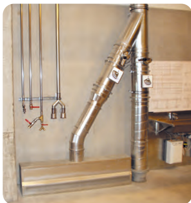
Dust extraction with an application specific pipe system
