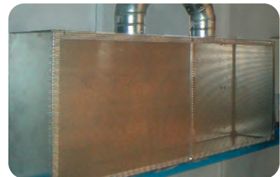
Extraction wall with perforated metal insert
