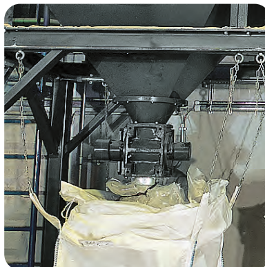
Removal through rotary valve
